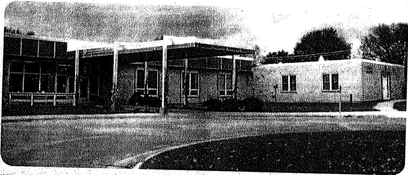
Lighting upgrades at the Algoma Medical Center & Long Term Care Unit are estimated to save 54,032 kWh annually.
