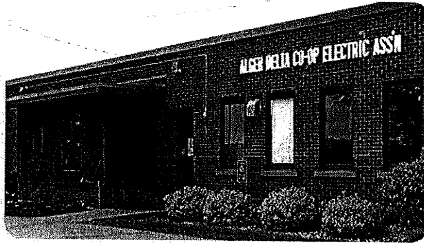
Alger Delta Cooperative Electric Association office facility.
