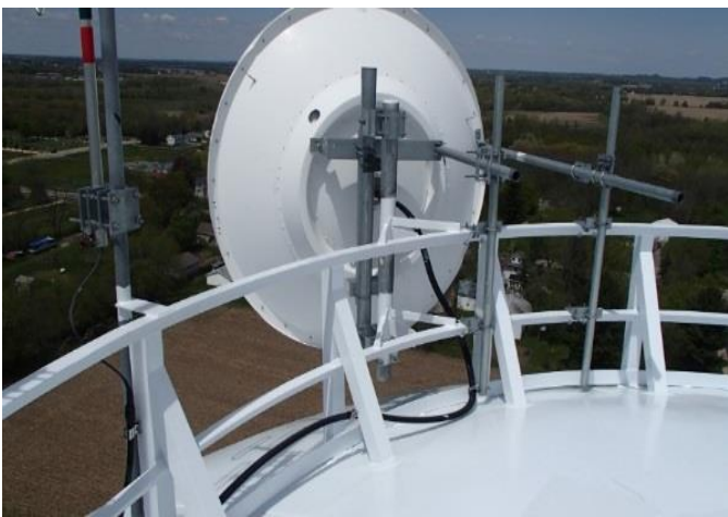
Exterior Coating Roof
