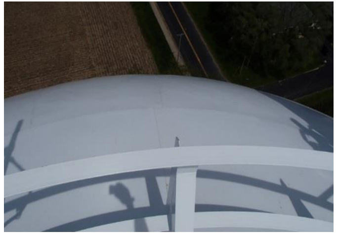
Exterior Coating Roof
