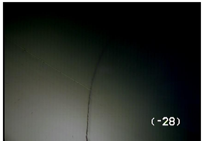
ROV Interior Coating
