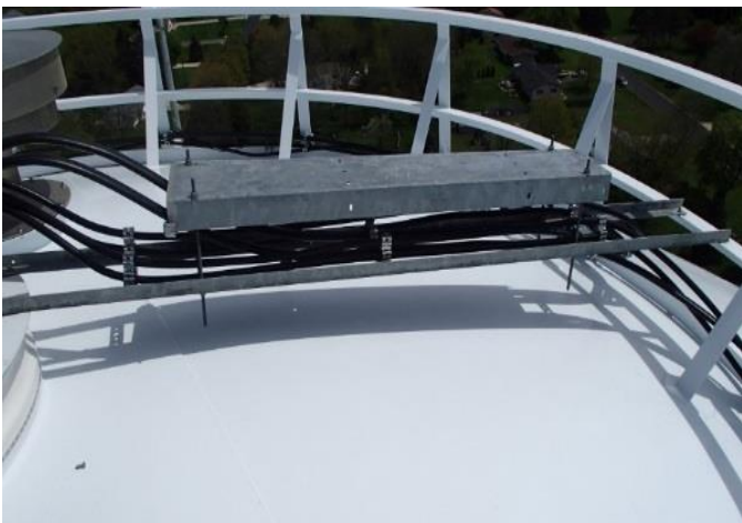
Exterior Coating Roof
