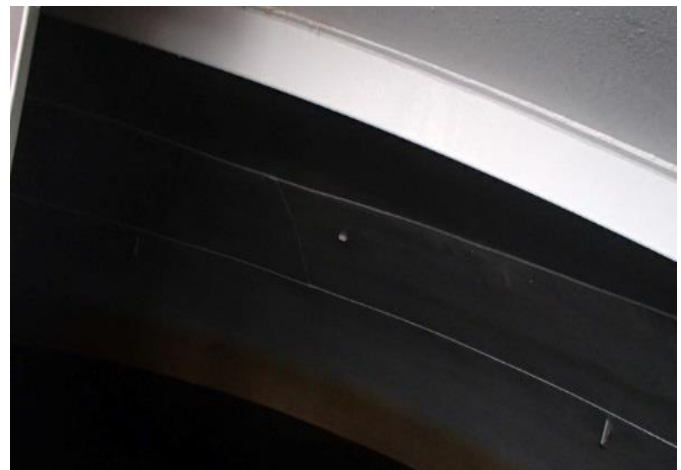
Interior Coating Roof
