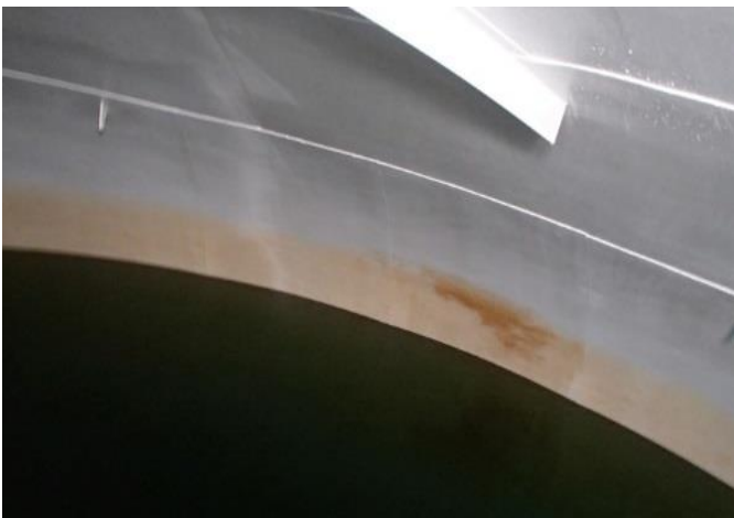
Interior Coating Roof
