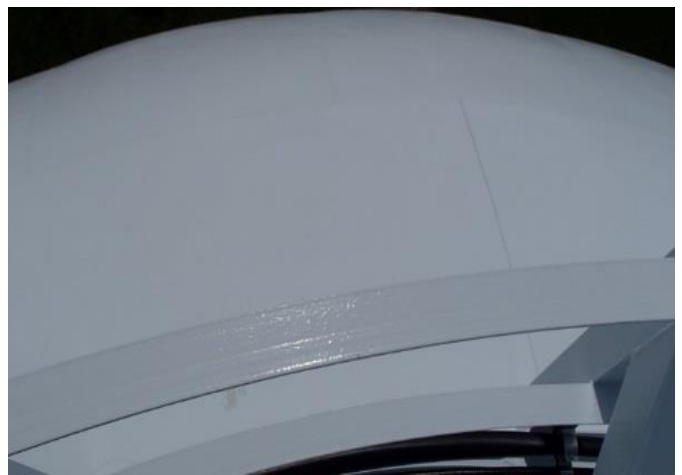
Exterior Coating Roof
