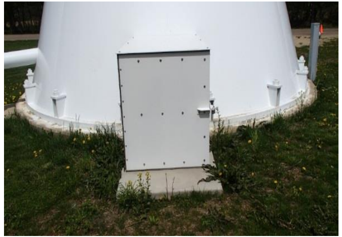
Exterior Base Structure
