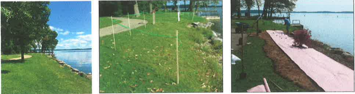
Site Preparation: Shoreline area before the garden, Marking the area, Killed grass, perimeter trench and paper weed barrier
