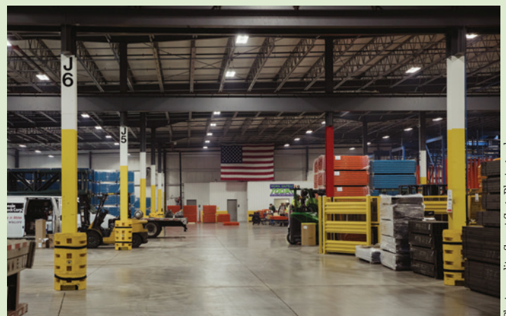
Stacked inventory inside the Steel King expansion
