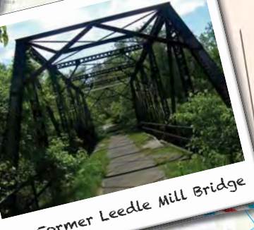
4. Former Leedle Mill Bridge
