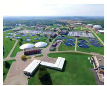
1. MMSD's Nine Springs Waste Water Treatment Plant
