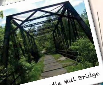
4. Former Leedle Mill Bridge
