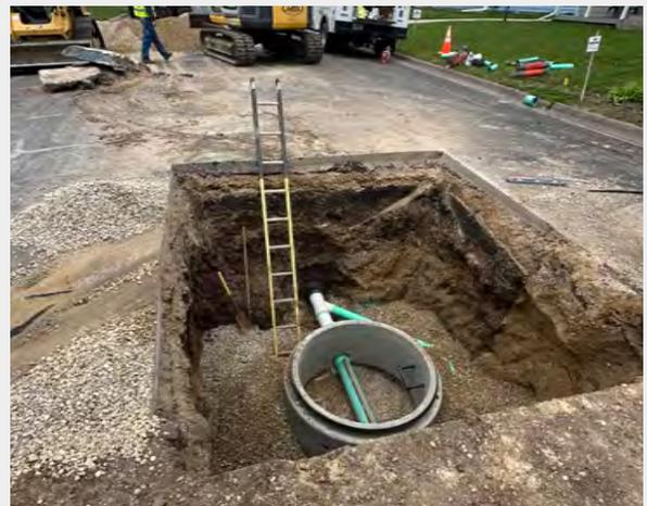
*Pictured: A sewer manhole being replaced on West Street after it had started to collapse. It was originally installed over 60 years ago.*
