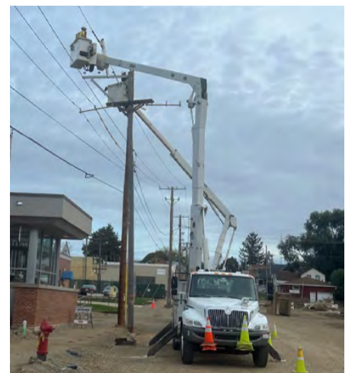
Pictured: SU Lineworkers working to replace the utility pole in front of the Administration office. Photo courtesy of Jill Weiss
